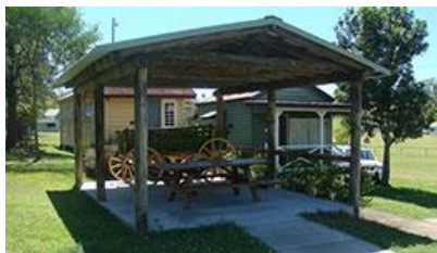
Shelter Shed with restored German wagon.
